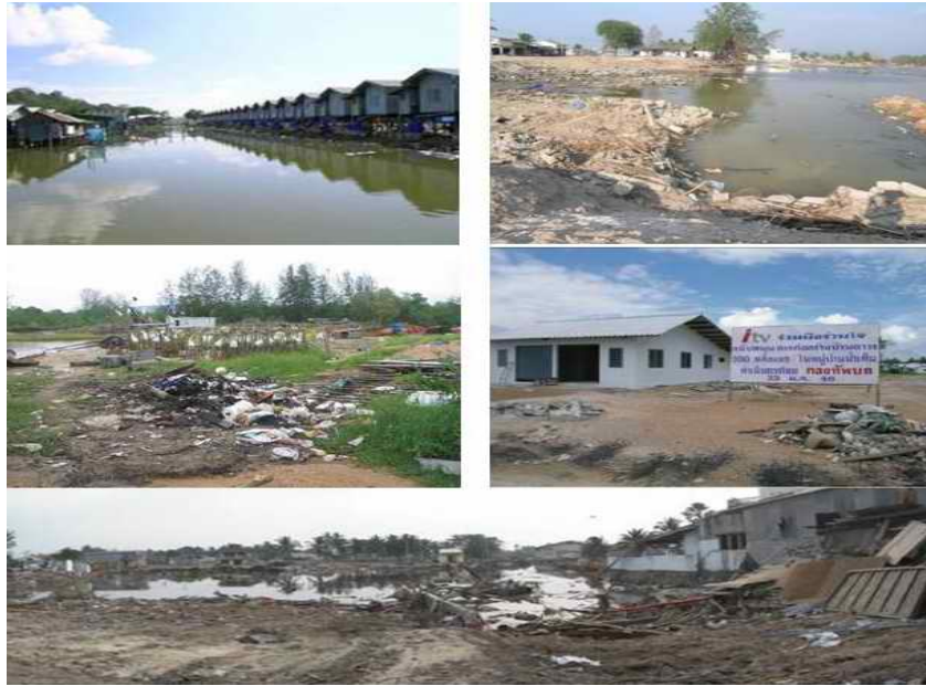
Picture 16: The assistance from the government by many houses without the sewerage system also contaminated the fresh water ponds.
